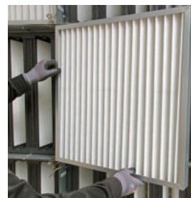
Easy replacement of pre- and main-filter
