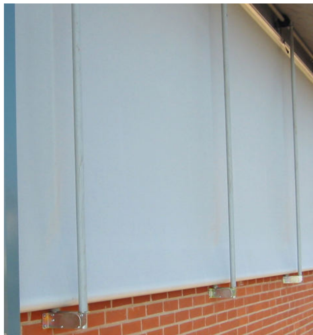
MSC wind protection pipes set
