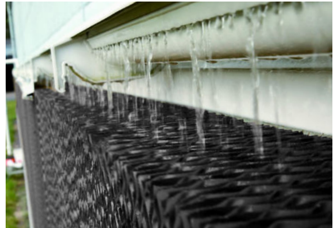
Water distribution in the Pad-frame system
