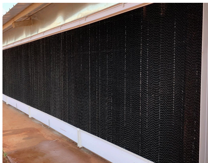
Munters Plastic Gutter (MPG) с система CoolPad RCP 150
